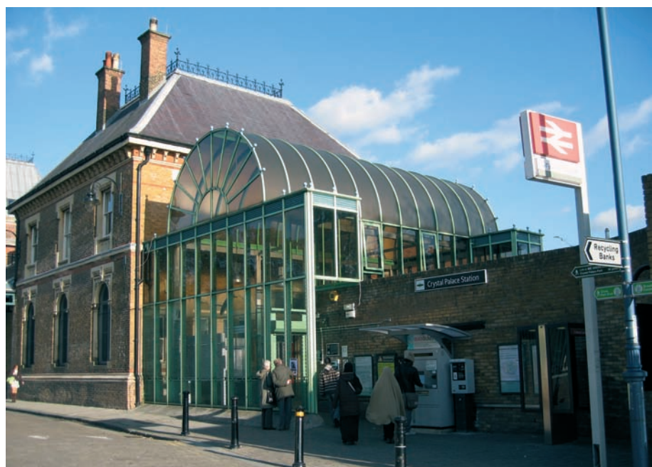
the modern railway station at Crystal Palace, formerly known as the Low Level Station (photo by Tim Locke)
